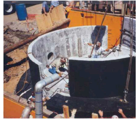
3. The second half of the sulfur pit being assembled with the first half.
