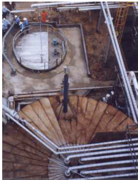
5. Completed sulfur pit from an aerial view
