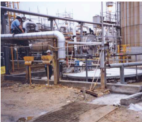
4. Completed sulfur pit from a ground view
